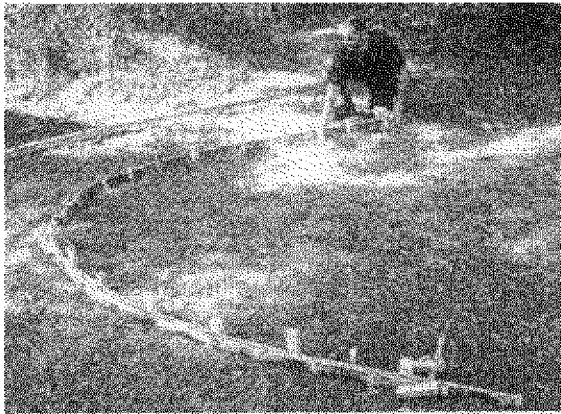
15-7 Construction of the arc with split bamboo
