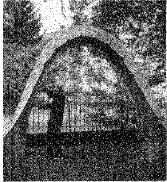
15-8 and 15-9 Earthquake resistant vault reinforced with bamboo FEB, Kassel, 2004
