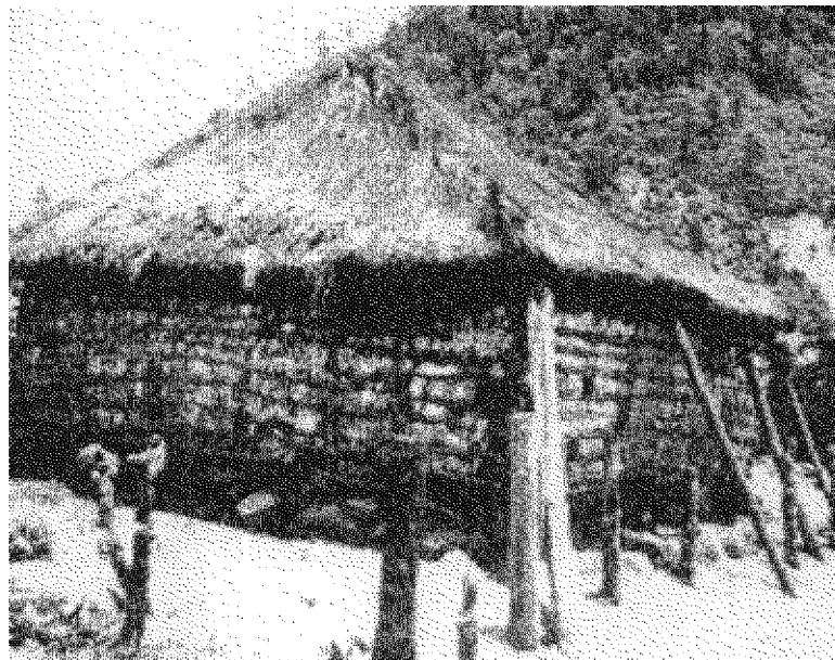
5-2 Wattle and daub structure, after a heavy earthquake in Guatemala (Minko, 2000)
