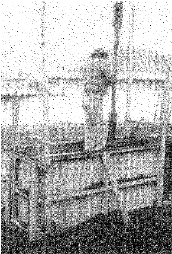
6-2 Tamper with two «heads», used in Ecuador (Minke 2001)
