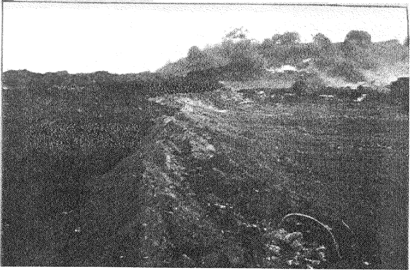
Plate 4. Barrier built to prevent the spreading of a lava flow at Kapoho, Hawaii, in January 1960. The wall is about 6 meters high. Lava is confined to the left of the wall. Eventually a new outbreak on the right of the wall flooded that area with lava also.
