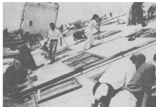
A Toppling over 4-Story Reinforced Concrete Apartment at Kawagishi in Niigata City ("Record of the Niigata Earthquake", Niigata Nippo, 1964)
