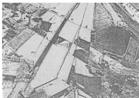
Destroyed Elevated Bridge at Highway Intersection (Robert Lacopi, "Earthquake Country", Lane Publishing Co., pp.138)
