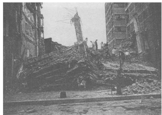
A Collapsed Building like a Sandwich (Earthquake Mexico '85'. The Munich Reinsurance Company, 1986)
