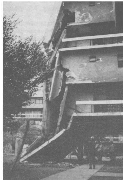
Collapsed Piloti of Reinforced Concrete building in Santiago City. By courtesy of Prof. Shibata.
