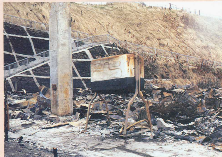
Ruins of fire; only chimney and kerosene tank standing; staircase for emergency climb up cliff
