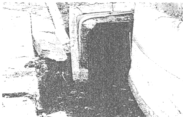
Photo 3 Aqueduct in Higashinada Wastewater Treatment Plant (Aqueduct is broken at a joint.)
