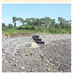
erecting low-cost but stable bank reinforcements. The plentiful rocks in the river bed were assembled into blocks with wire netting and fastened to the banks in tiers.
