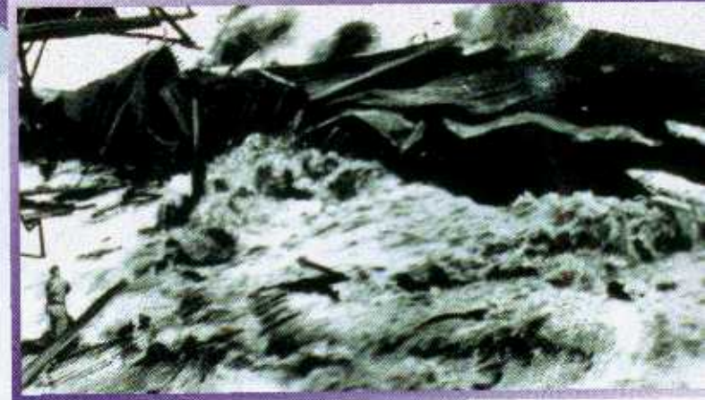
Hilo Harbor, Hawaii, April 1, 1946, Aleutian Islands earthquake. Photo taken from the vessel Brigham Victory of tsunami breaking over Pier 1. The gentleman on the left did not survive. (NOAA)
