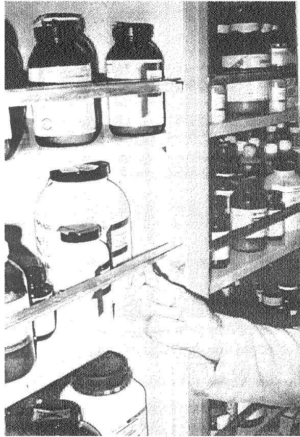
Figure 4-3 Brackets designed to keep lab chemicals on shelf, Rinconada water treatment plant. Photo taken after the 1989 Loma Prieta, Calif., earthquake.
