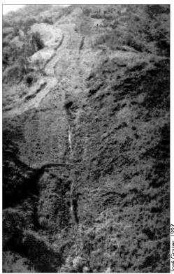
Pipelines located on slopes are exposed to breaks and deformation because of slow moving landslides (creep) and sudden collapse of slopes.
