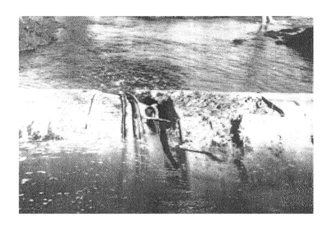
FIGURE 2-3 Aqueduct Damage During 1979 Guerrero Earthquake
