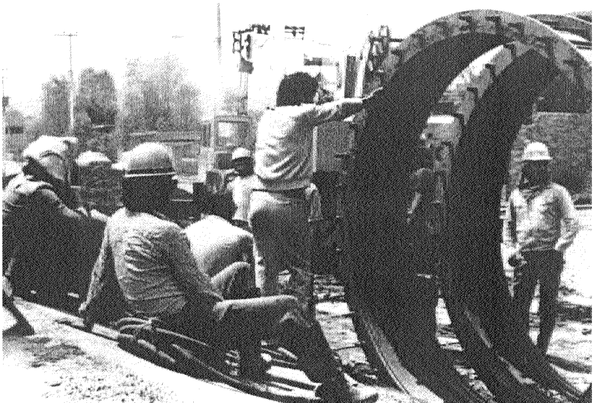
FIGURE 6-12 View Of A Steel Repair Saddle
