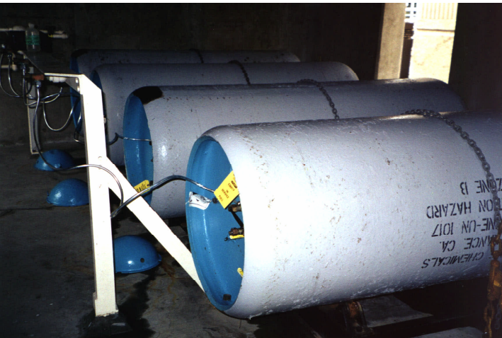
21 Chlorine Tanks (Photo courtesy Moulton Niguel Water District)
