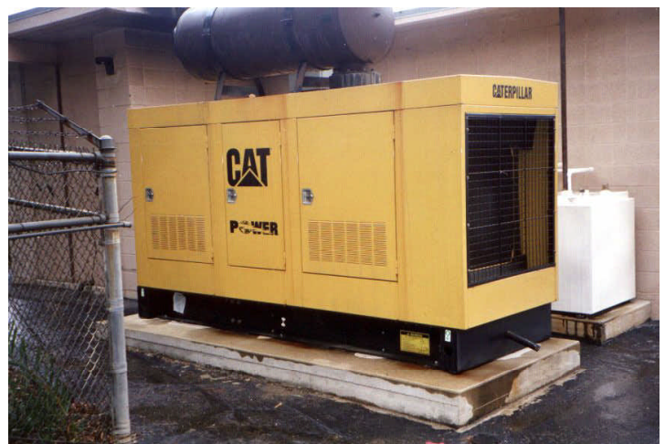
24 Emergency Generator Detail (Photo courtesy Moulton Niguel Water District)
