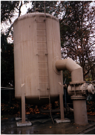
31 Vertical Vessel - Surge Tank (Photo courtesy Moulton Niguel Water District)
