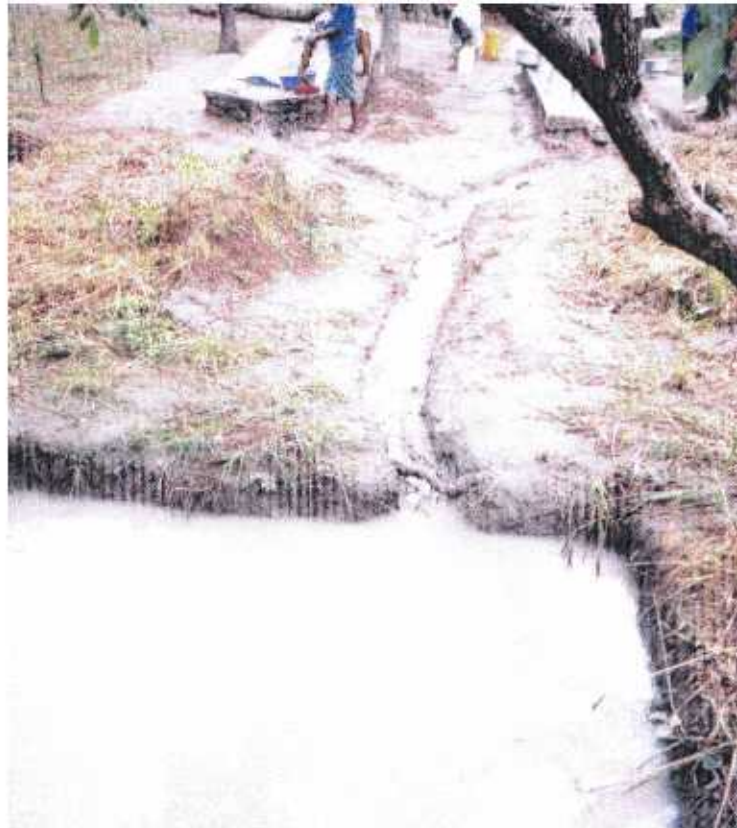
Poorly designed soakpit, Tanzania
