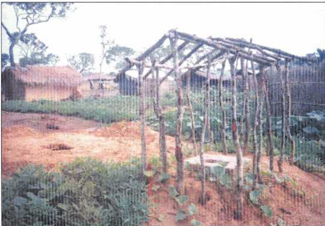
Family pit latrine under construction
