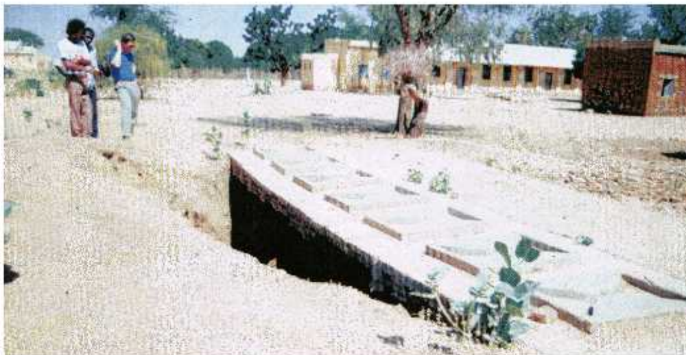
Failed unlined trench latrines, Sudan
