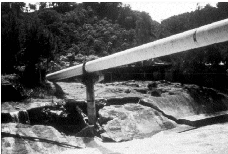
Flood damage to the bridge supporting the main water pipe of the Oroquieta system in Costa Rica in October 1999. Some 500 tons of concrete were displaced.
