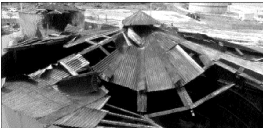
Damage to the roof of a water tank sustained during a hurricane.
