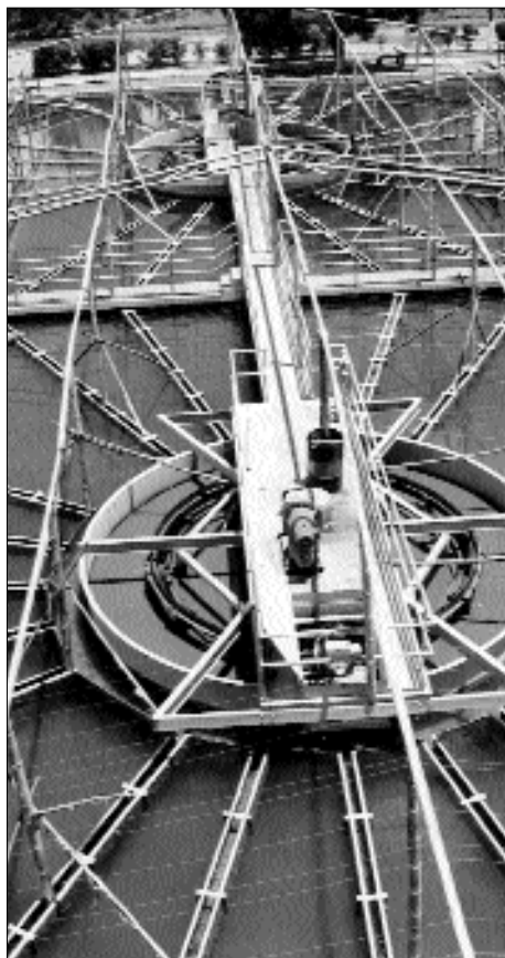
As an emergency measure during the eruption of the Pichincha volcano in Ecuador, in 1999, temporary coverings were installed to protect the water treatment plant from ash-fall.
