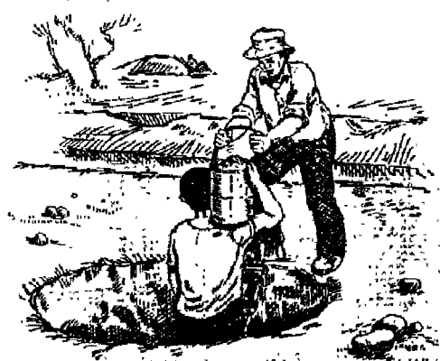
Figure 4: Digging an infiltration well
