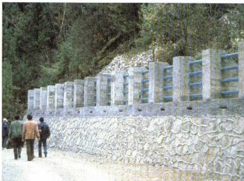
Flood and slide barrier on road Jiuzhaigon, China.
