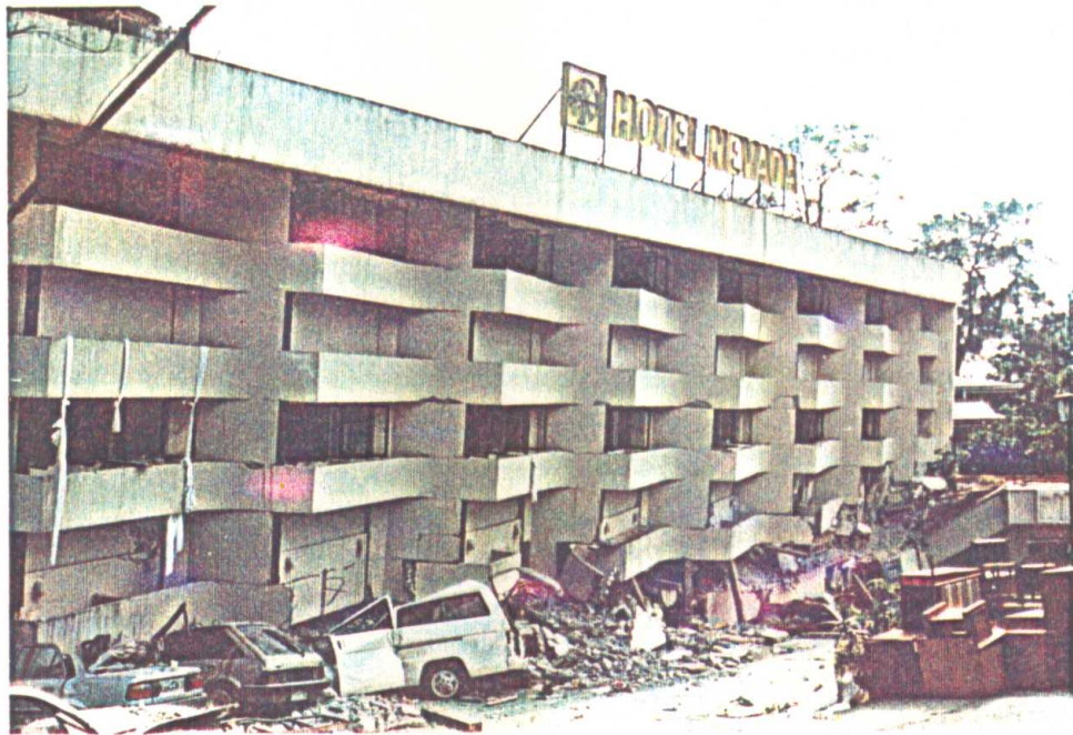
Photo 3.5 Failure of Hotel Nevada, 5-storey r.c. building ground floor collapsed. Typical irregular and brittle structural system with inclined walls exhibiting failure or heavy damage in other earthquake in the world (Montenegro, Yugoslavia earthquakes 1979, El Asnaw, Algeria earthquake, 1980).
