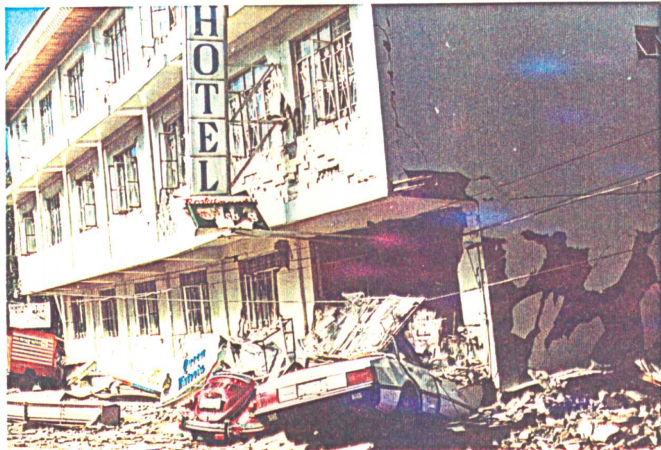
Photo 3.6 Hotel Queen Victoria 3-storey r.c. building with pronounced cantilivers. Typical high intensity vibrational effect producing intensive nonstructural and partial structural damage.
