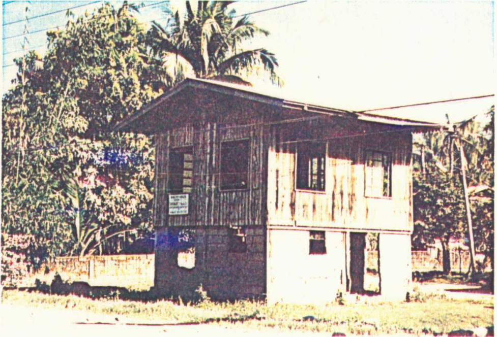
Photo 4.6 Typical village timber house with brittle and not integrated ground floor of block masonry. Damage and failure could be expected at large earthquake intensities.
