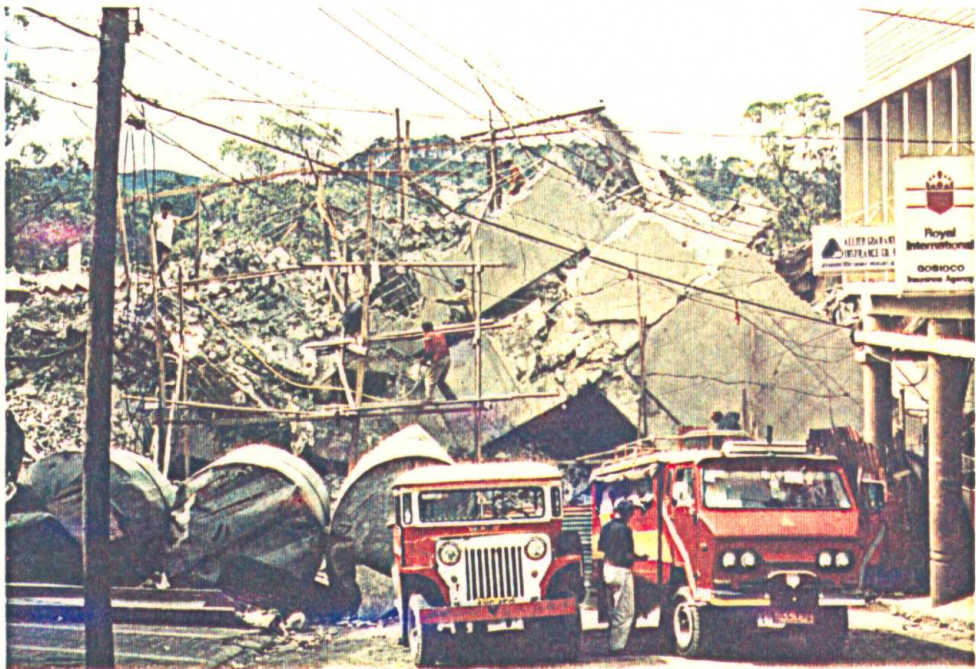
Photo 4.11 Failure of seven story Park Hotel in Baguio City constructed as r.c. frame structure with brittle and non-adequate proportioning of column and beam sections.
