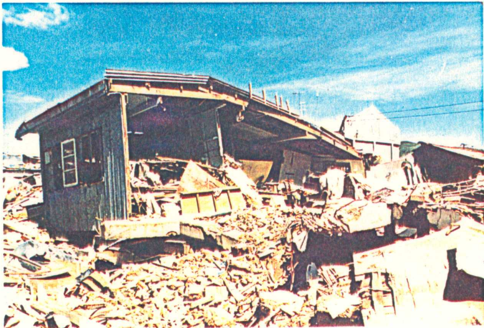
Photo 4.9 Few timber framed houses collapsed due to the vibrational effects of the earthquake, but some were damaged by the collapse of neighboring r.c. buildings as shown here. (Baguio)
