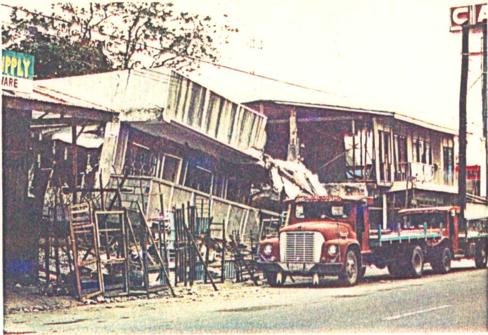
Photo 4.8 Reinforced concrete framed houses (non-engineered construction) performed poorly in comparison with timber framed houses - here (Agoo) an r.c. structure has collapsed between two lightly damaged timber framed structures.
