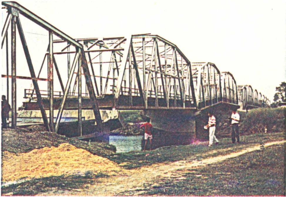
Photo 4.18 Failure of Carmen Bridge on the road Manila-Baguion, out of 12 spans, 6 collapsed or experienced large deformation due to liquefaction causing intensive settlements and tilting of piers. Sandboils due to liquefaction observed in the vicinity of the bridge.
