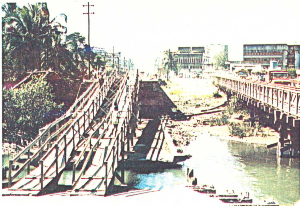
Photo 4.20 Failure of the bridge over Pantal River in the central business district of Dagupan City, due to liquefaction causing failure of piers and abutments. Left temporary walkway and failed bridge deck, right temporary Bailey Bridge.
