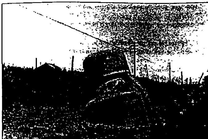
Photograph 2-3. Floating manhole as a result of liquefaction following Nigata earthquake.
