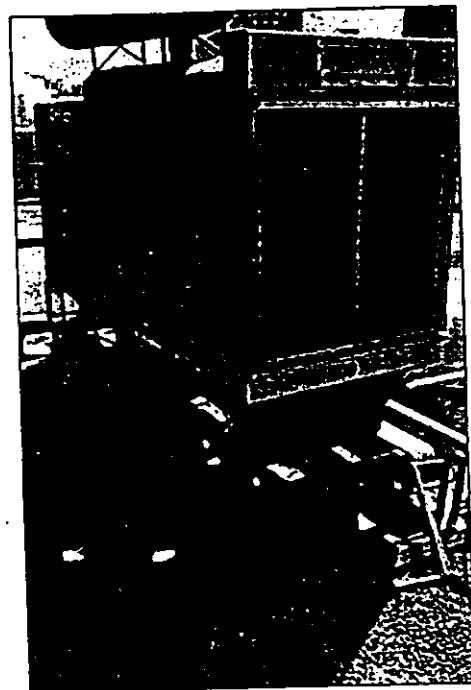
Photographs 3-32, 3-33, and 3-34. Spring vibration on emergency generator damaged in Whittier earthquake.
