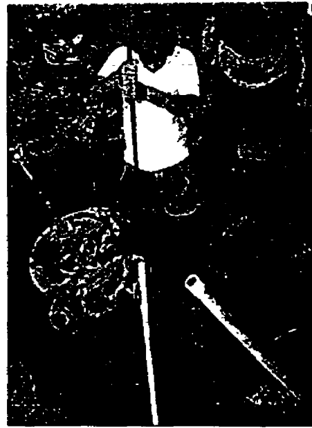
Photograph 3-8. Well casing bent 15 degrees from vertical as a result of lateral spreading in Dagupan, Philippines.
