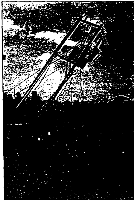
Photographs 3-60 and 3-61. Unanchored pole platform transformer toppled in Erzincan, Turkey. Pole with transformer toppled as a result of liquefaction at its base in Costa Rica.
