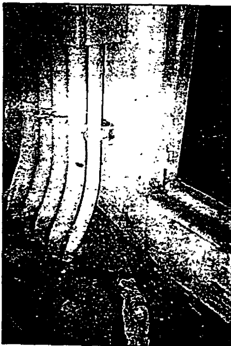
Photograph 3-25. Cracking from differential ground settlement around pipe-supported treatment plant structure.
