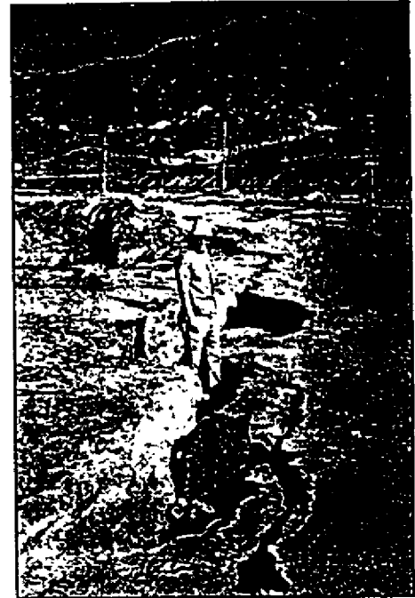
Photograph 3-10. Ground cracking above clearwell.
