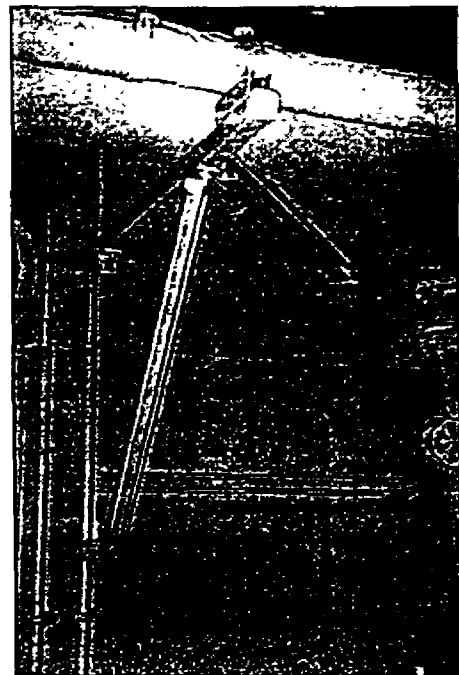
Photograph 3-27. Pipe support providing support in three orthogonal directions.
