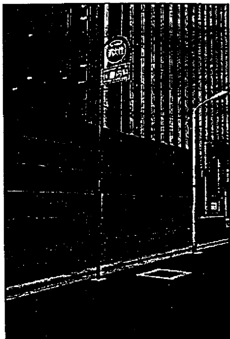
Photograph 3-78. Sign on pole marks below grade fire hydrant in Tokyo, Japan.
