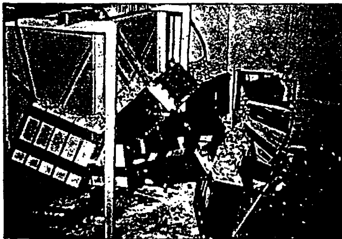
Photograph 3-66. Unanchored batteries topple.
