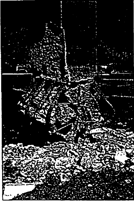
Photograph 3-73. Non-ductile concrete column failure in San Fernando.
