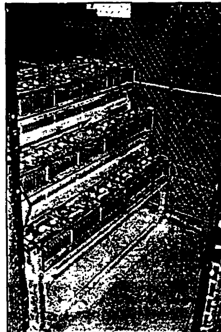
Photograph 3-67. Battery rack with restraint design weathered Loma Prieta earthquake at Rinconada Water Treatment Plant.
