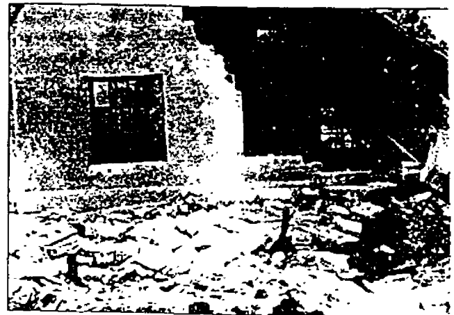
Photograph 3-72. Partially collapsed unreinforced masonry building
