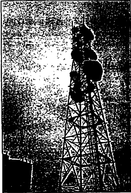
Photograph 3-69. Microwave radio system remained operable following Erzincan, Turkey earthquake.
