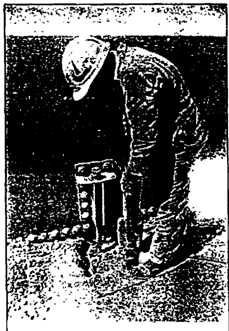
Photographs 3-101 and 3-102. Stretched anchor bolts on tanks following San Fernando and Seattle earthquakes.
