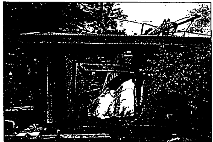
Photograph 3-105. Elevated tank collapsed through the police station in Umingan, Philippines.
