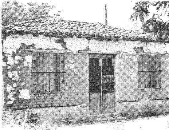
Poorly constructed adobes experienced moderate damage
