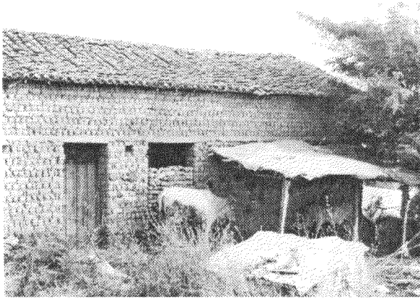
Well constructed adobes experienced no damage at all
