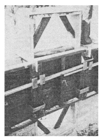
Shows the joint between two modular forms with the metal tube keeping them in line. The door frame occupies exactly one form as is the case with a window frame. Notice the bracing of the door frame.
