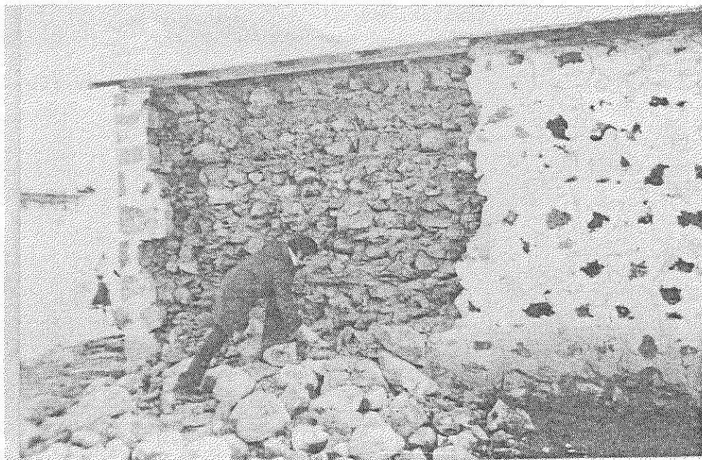
FIG. 4 INADEQUATE BOND BETWEEN TWO STONE LAYERS ( March 1976 , Susuz Earthquake , Turkey )
