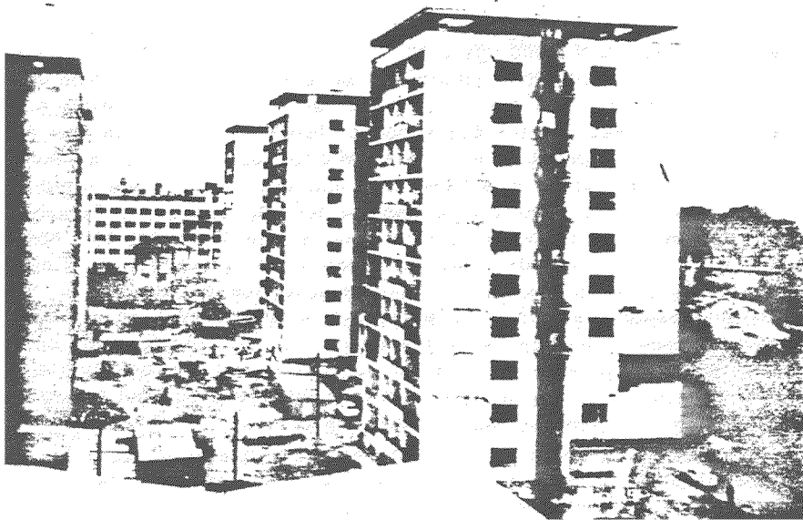
Damages to high rise building in Skopje (Yugoslavia) earthquake of July 26, 1973
