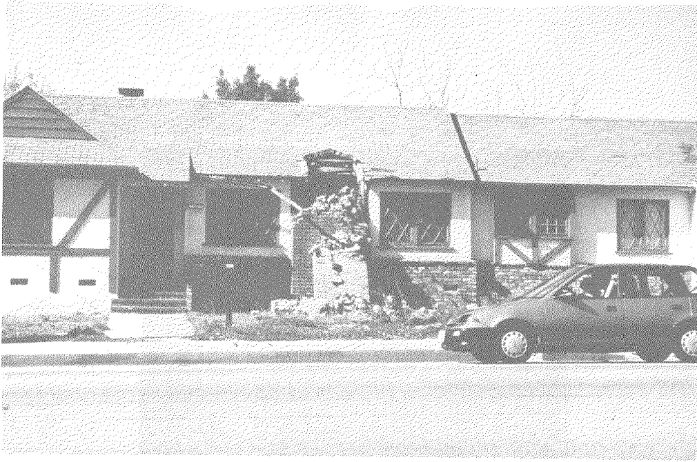
Fig. 42 Failure of a masonry chimney.
