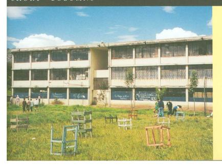
Two common structural deficiencies are "soft" stories (such as stories without infill walls) and "short" columns (columns effectively shortened by partial infill walls). Shown are examples of each in Quito schools, and an earthquakedamaged building that had a "soft" first story.
