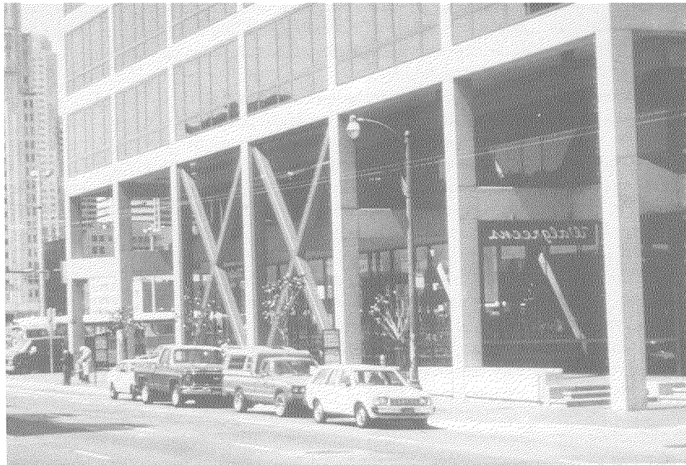
(1) Overview of building: the steel braces were used for lateral stiffening of the original RC building
