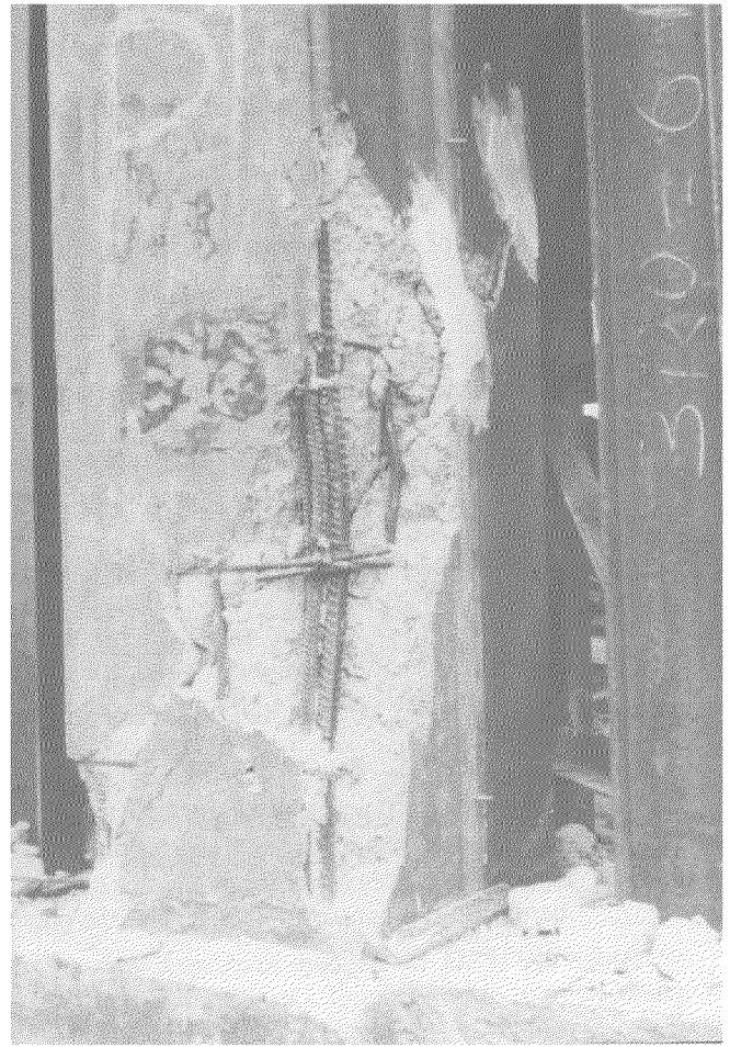
48 (b) Shear failure of the 1st-story column
