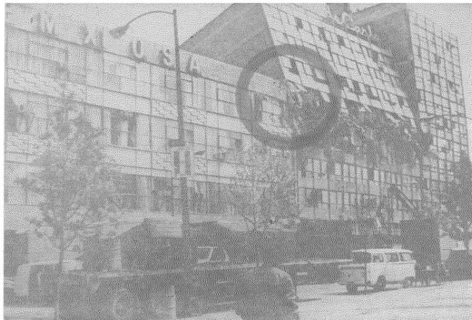
Fig. 24 COLLAPSE OF TWO INTERMEDIATE STORIES DUE TO HAMMERING OF ADJACENT BUILDINGS
