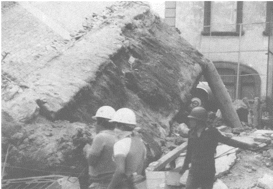
Fig. 23 (b) Close-up showing pullout of friction pile
