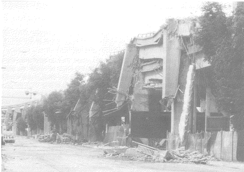
Fig 33 (b) The part that collapsed
