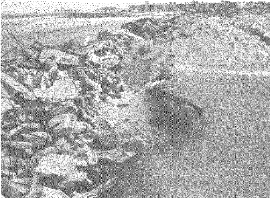
Flood and erosion-damaged road, St. Augustine, Florida.
