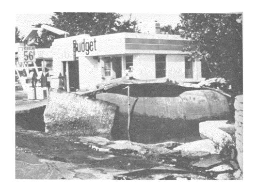
Empty gas storage tanks, Austin, Minnesota. During floods, gasoline and propane tanks may float free, causing fire and pollution problems as well as increased flood damages.
