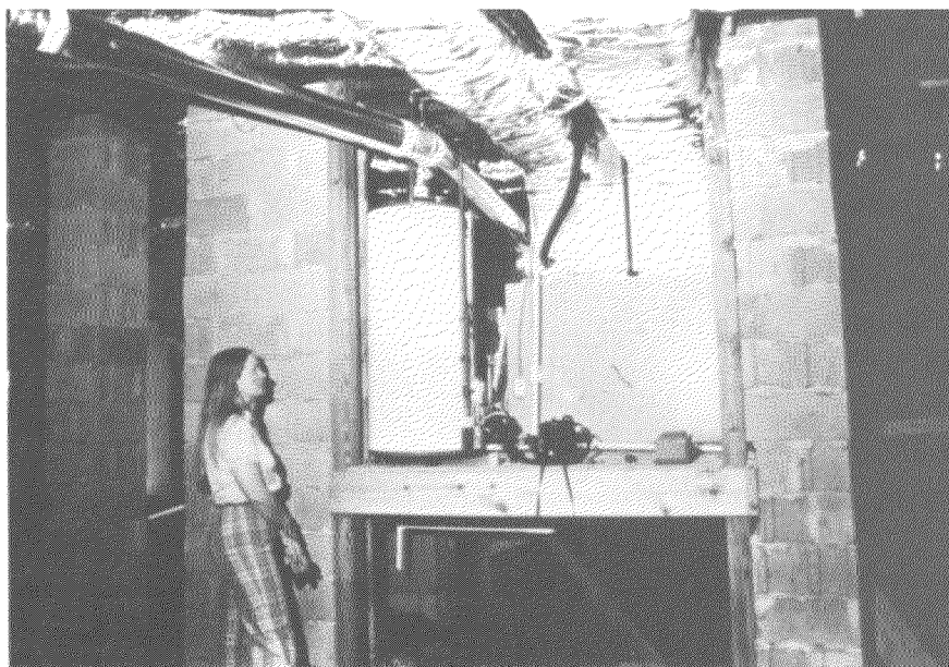
Water heater elevated on platform
