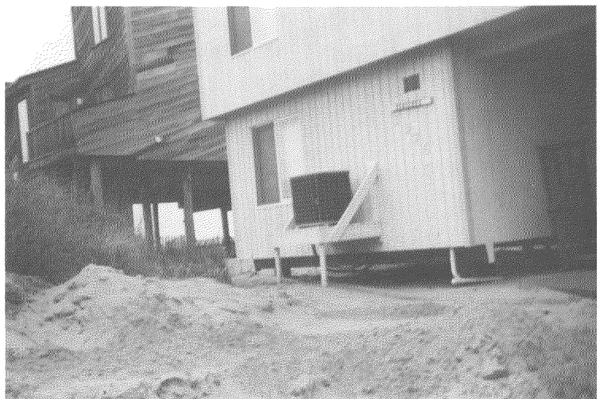
Air conditioning unit on raised platform
