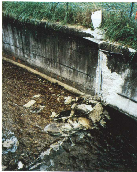
Photo 2 Damaged concrete wall of drain
