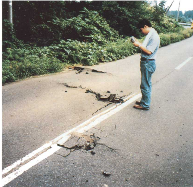
Photo 3 Buckled pavement
