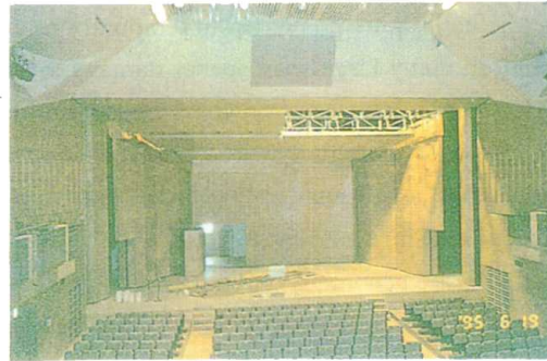
fig.3 Fallen acoustic boards
