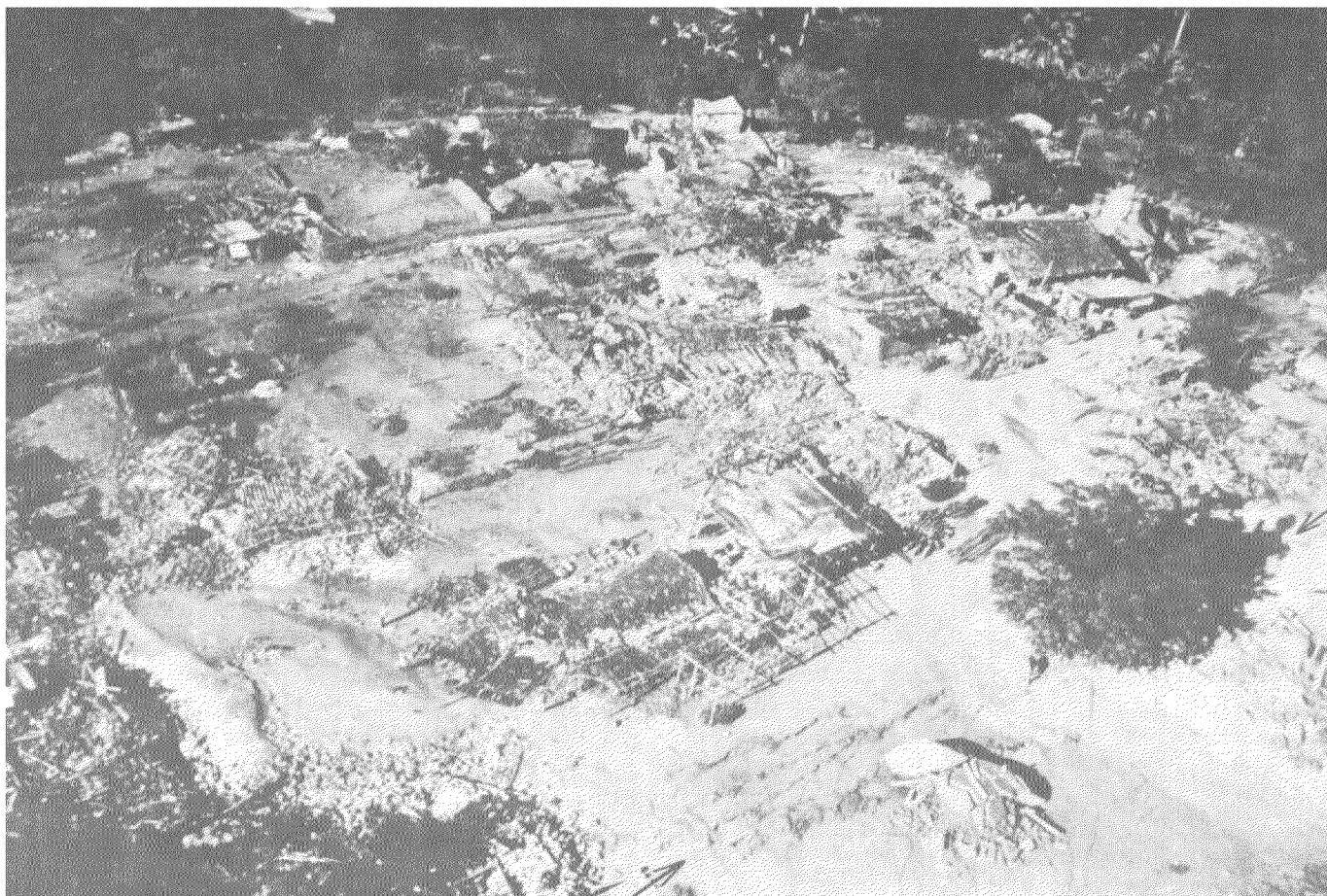
FIGURE 28.—Part of the village of Subinal, 7 km west of El Progreso, showing the destruction of adobe structures near the Motagua fault trace. The fault is a broad zone of ground cracks that cuts diagonally across the lower right corner of the photograph (arrows).
