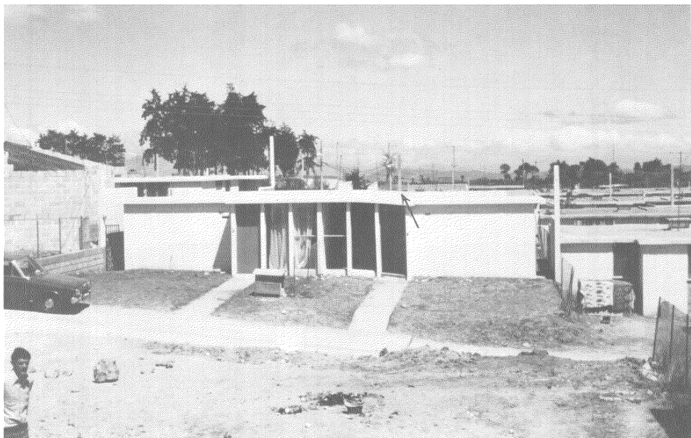
FIGURE 31.—Fault damage to a house in Guatemala City. The roof, foundation, and sidewalk have been displaced vertically.
