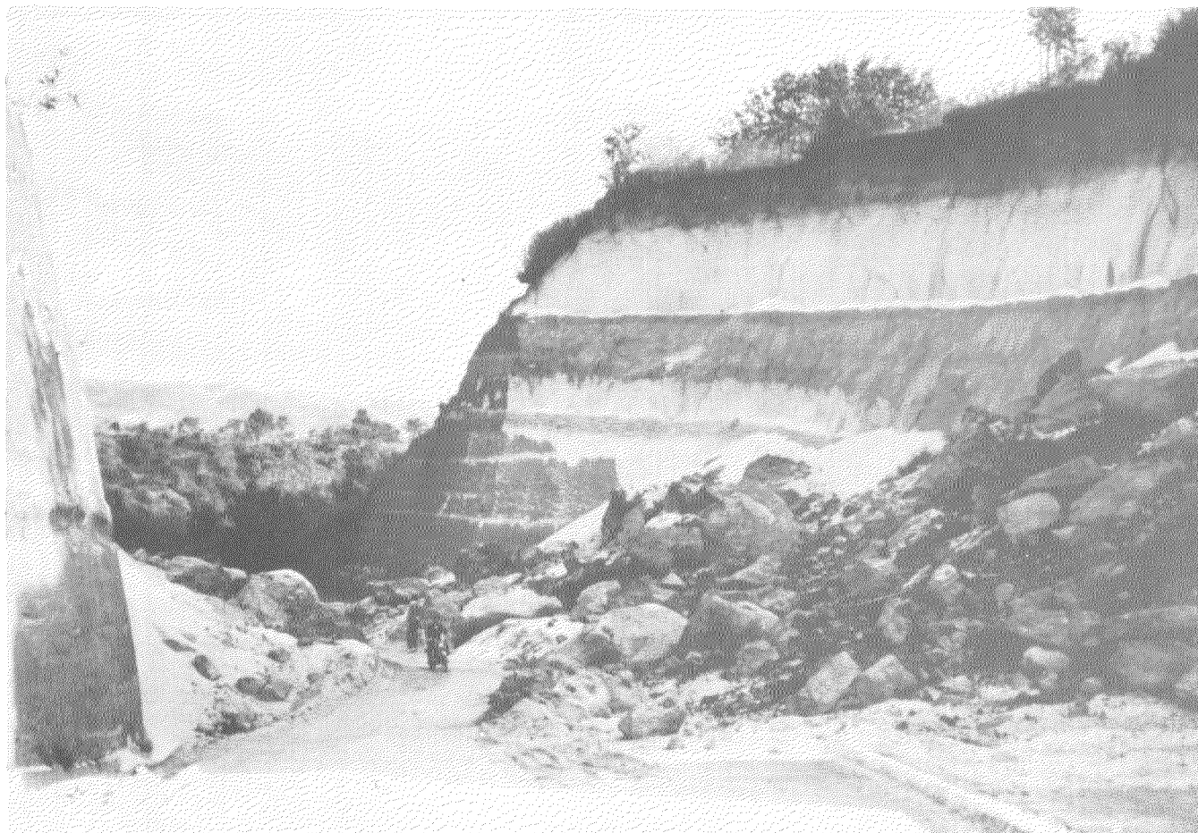
FIGURE 34.—Landslides in steep road cut in stratified pumice and ash deposits at San Cristobal, west of Guatemala City.
